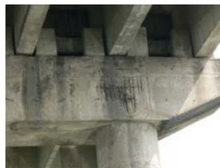
21#墩盖梁锈胀露筋
